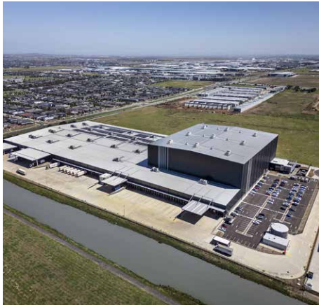
FIGURE 4 LANDMARK CONSTRUCTION PROJECTS
